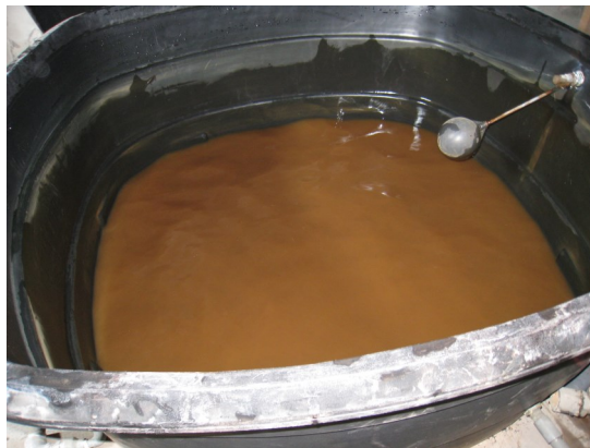
Contaminated Cold water tank
